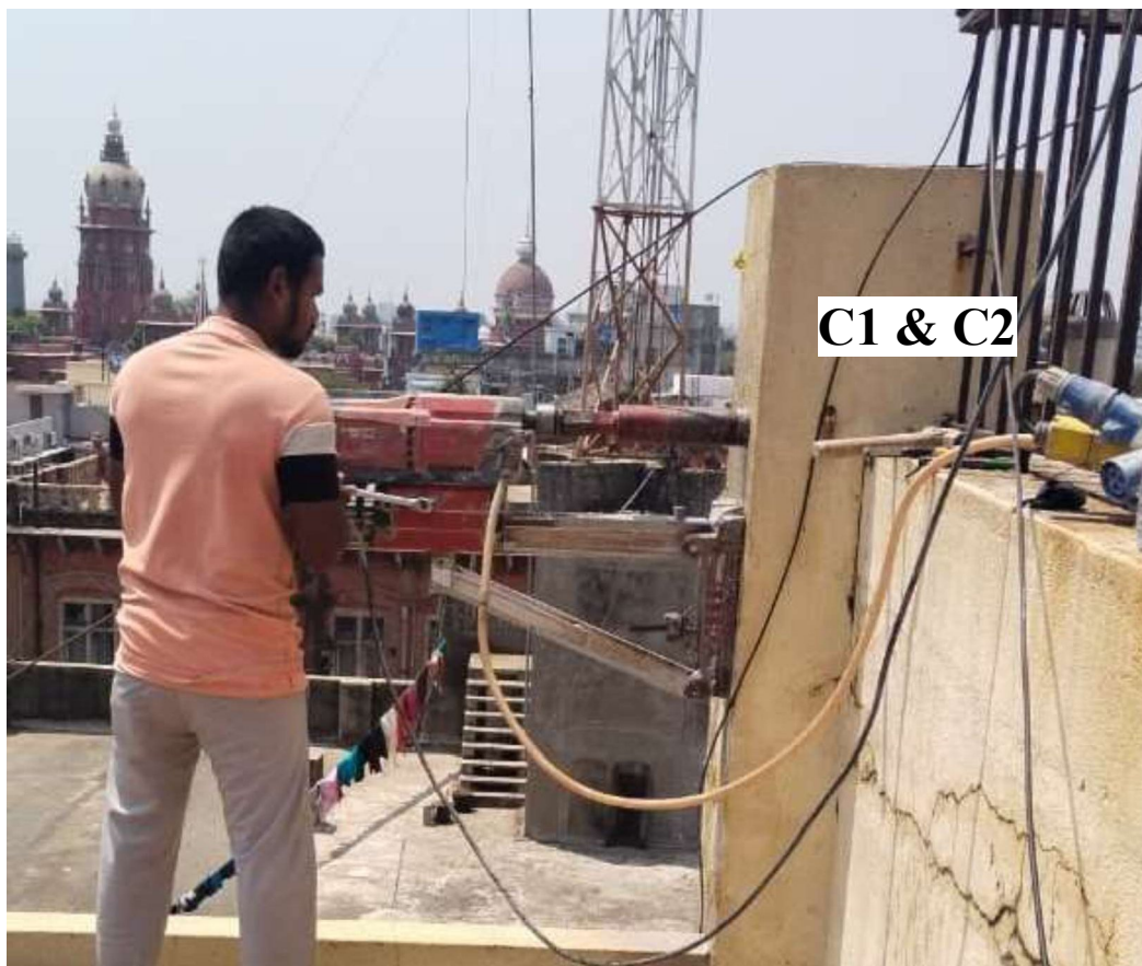
Figure.3 Core drilling at C1 and C2 locations
