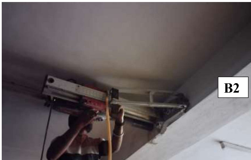
Figure.6 Core drilling at (a) C7 (b) B2
